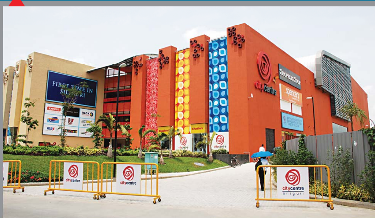
Front View of Mall & Office Building - City Centre , Siliguri
